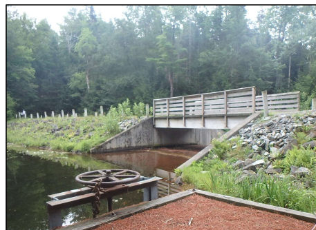
Lowell Lake Dam, Londonderry
