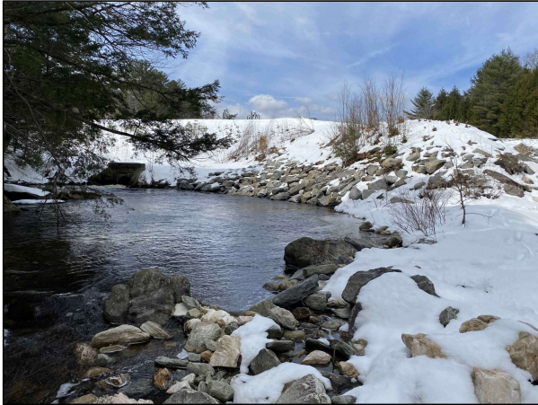
Gale Meadows Dam and Dike, Londonderry
