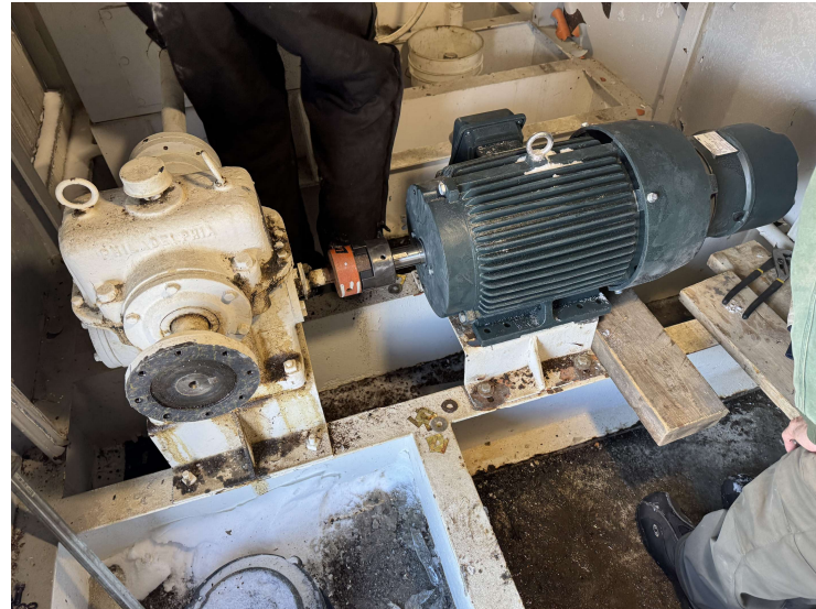
Gate 3 – new motor with integrated braking system, January 2026
