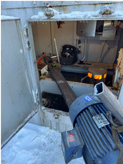
Gate 3 – Removal of old motor, January 2026
