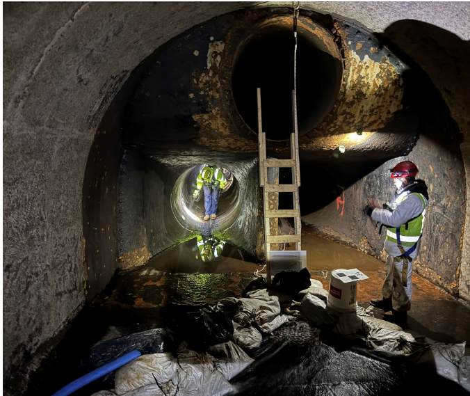
Tunnel to Penstock Transition post cleaning, December 2025
