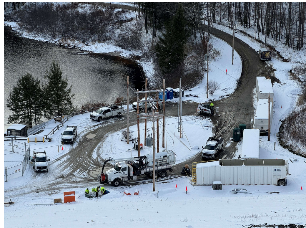
Penstock Cleaning Operations, Vector Trucks, wastewater tanks, etc., Waterbury Dam
