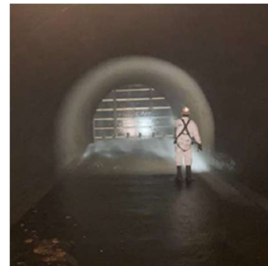
Waterbury Dam Head Gate in Closed Position, Fall 2024 prior to cleaning.
