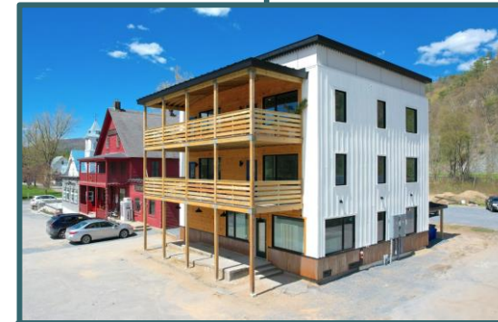
501 Main New $1.4m, 9-unit residential (half affordable, half market rate) and coffeeshop completed in 2023.
