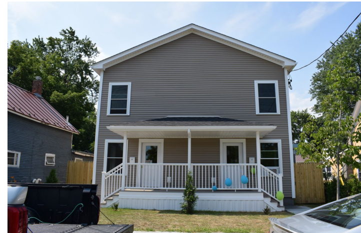
Lower photo: Completed home in Burlington
