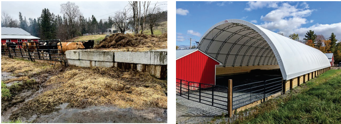
Figure 2. (Left) Uncovered barnyard had runoff issues in wet conditions. (Right) New covered barnyard area provides a clean area for manure storage and livestock and eliminates runoff concerns.
