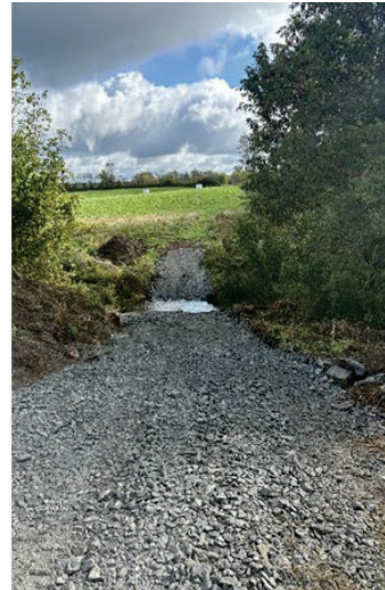
Figure 3. (Left) Trees and shrubs planted in the newly established riparian buffer zone. (Right) Stream crossing installed to enable livestock crossing with reduced impacts.
