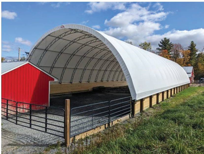
Figure 16: A barnyard improvement and cover was installed through the Best Management Practices (BMP) Program to reduce agricultural runoff to an adjacent stream from the farm's outdoor livestock area in the Connecticut River Watershed. Farms that are certified organic under the National Organic Program standards are required to ensure livestock have access to the outdoors every day. Covering those areas to prevent rainwater from mixing with animal waste can be an effective tool for reducing runoff and improving water quality on farms, especially during the winter months.
