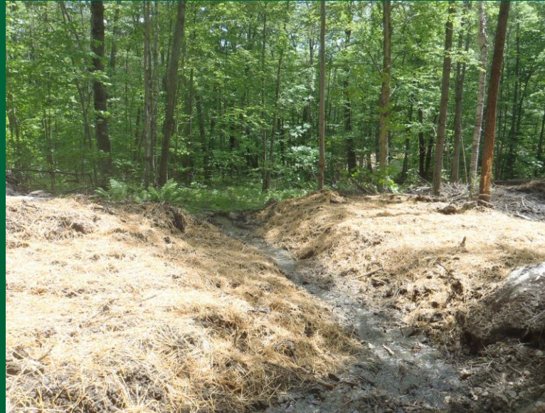
Prevent Soil Erosion
