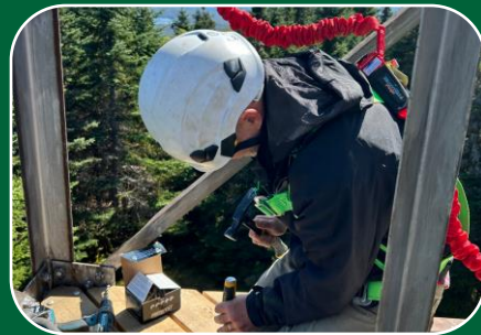
Restoring steps at fire tower
