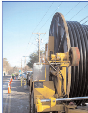
■ Pull and splice cable
