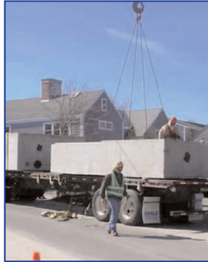
■ Installation of manholes
