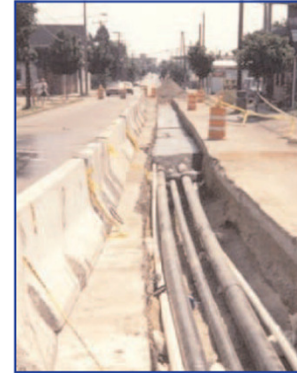
■ Lay conduit and encase in concrete
