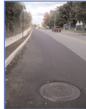
■ Final treatment with new asphalt
