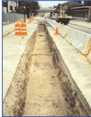
■ Mark location of line and dig trench
