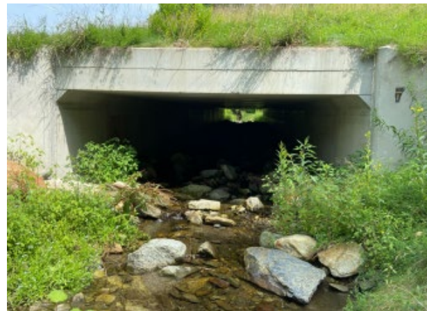
16' x 6' box culvert
