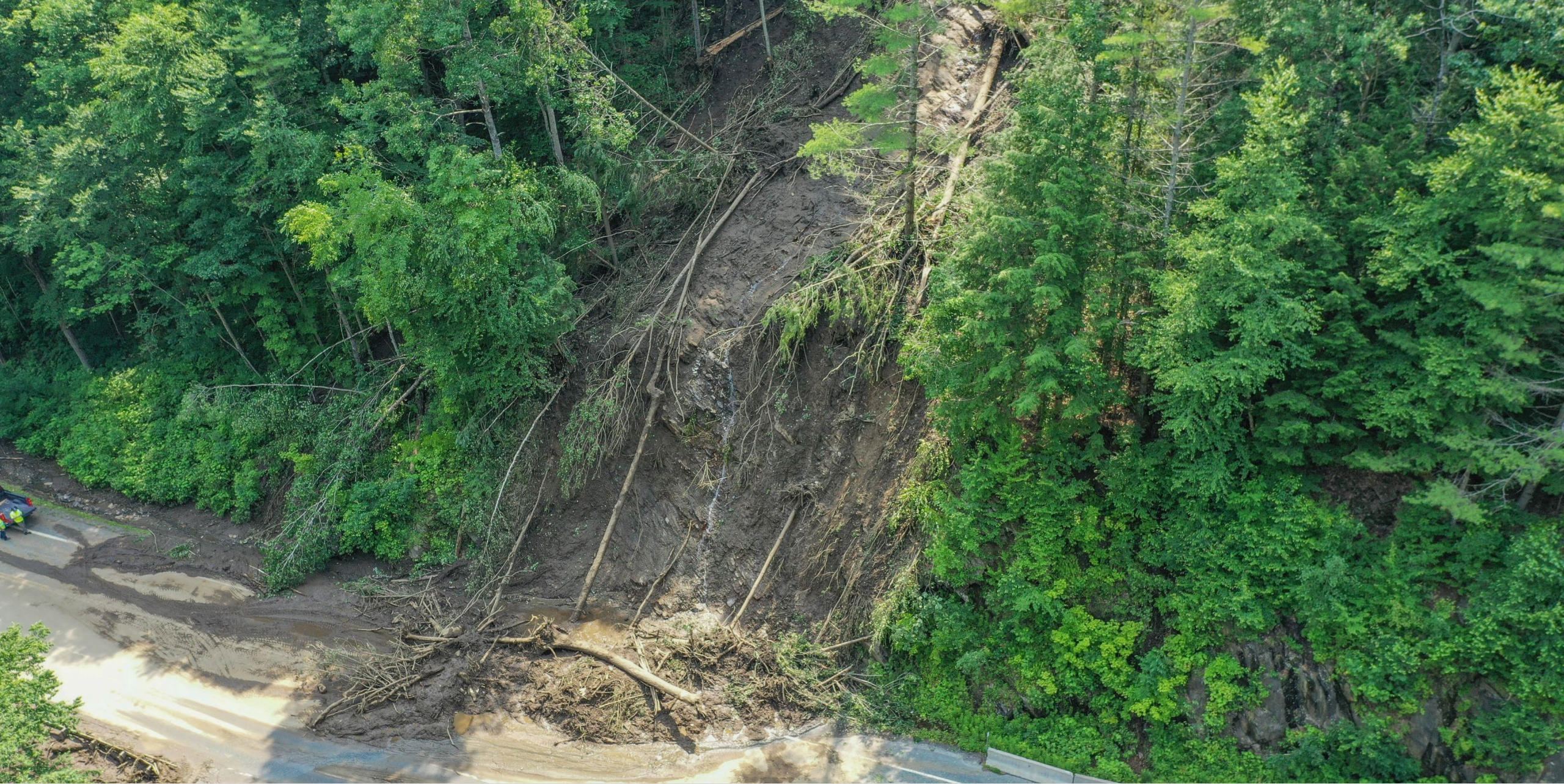
Reading VT106 Washout
