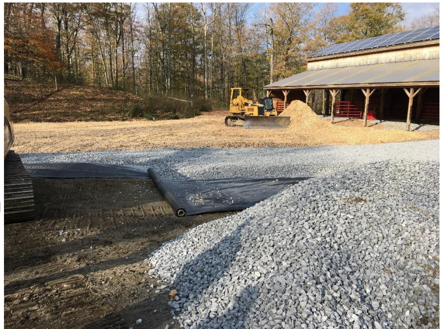
Figure 17. The Woodchip Barnyard Replacement project is a cost-effective solution to reduce water quality impacts from existing winter heavy-use areas and contains a drainage layer overlain by woodchips. The drainage system underneath collects and diverts the effluent to a collection system. The top layer of woodchips is replaced each year and can be composted and then field applied along with collected effluent. This project was funded by the Agency of Agriculture, Food and Markets through Water Quality Grants to Partners and Farmers.
