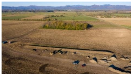
Figure 20. A wastewater disposal mound is a soil absorption system placed above the natural surface of the ground. The town of Addison installed a community wastewater disposal mound system to treat municipal waste in June 2019. The project was financed by the Clean Water State Revolving fund.
