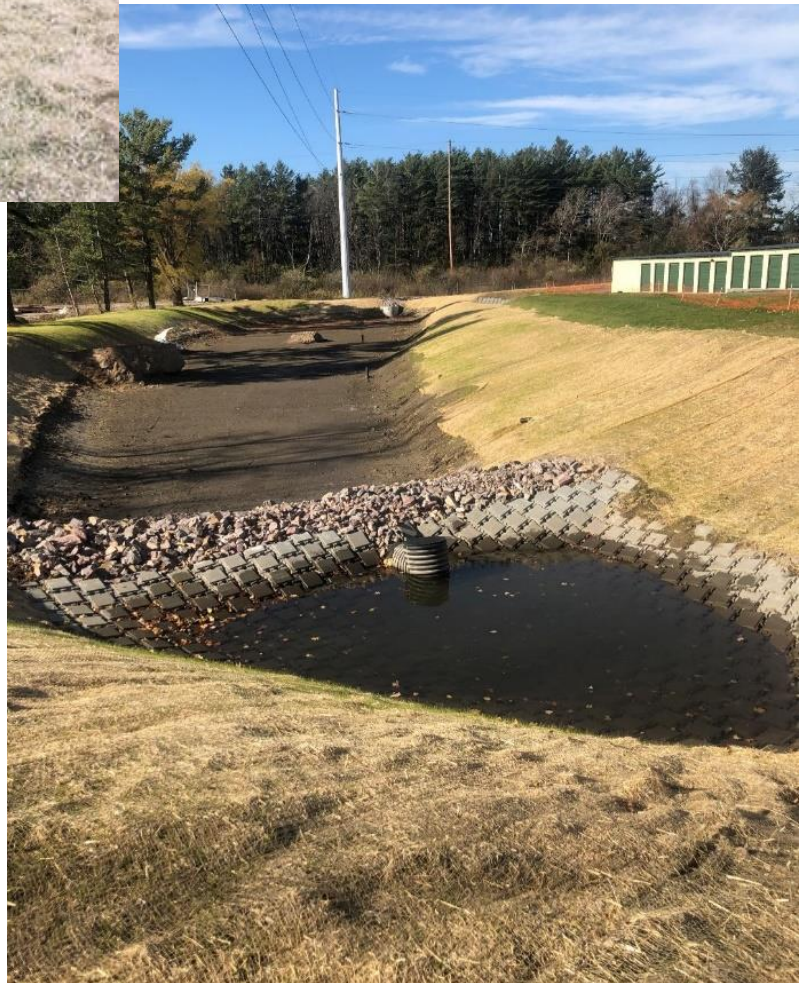
Figure 19. This constructed wetland before (left) and after (below) was installed along a right of way in Shelburne, Vermont and provides stormwater treatment for approximately 39 acres of impervious surfaces including two sections of Shelburne Road. This stormwater treatment practice was completed in May of 2021.
