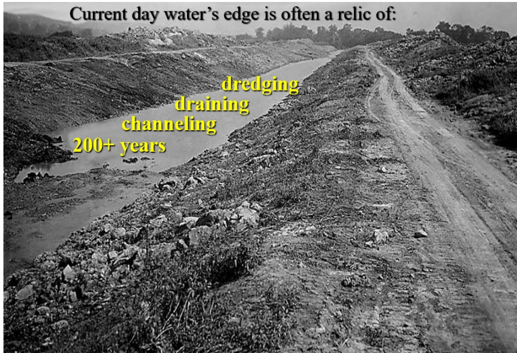
Figure 1: Many of Vermont's rivers are still unstable and recovering from past practices
