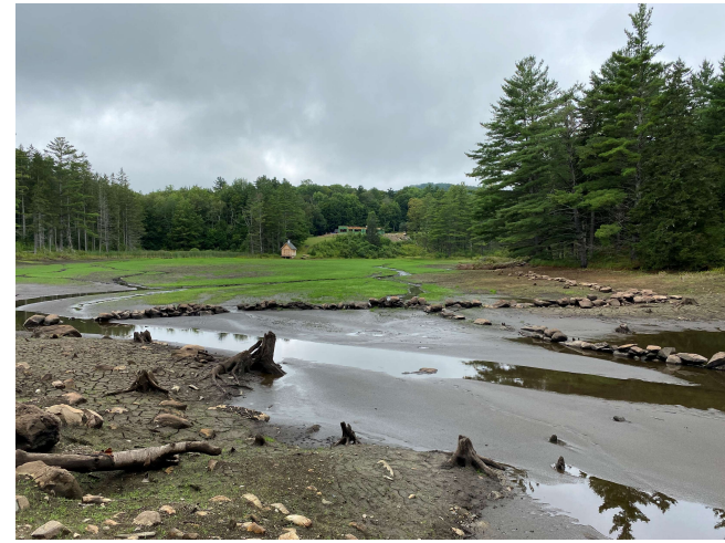
Lyons Pond Dam, Peru, LOW Hazard
