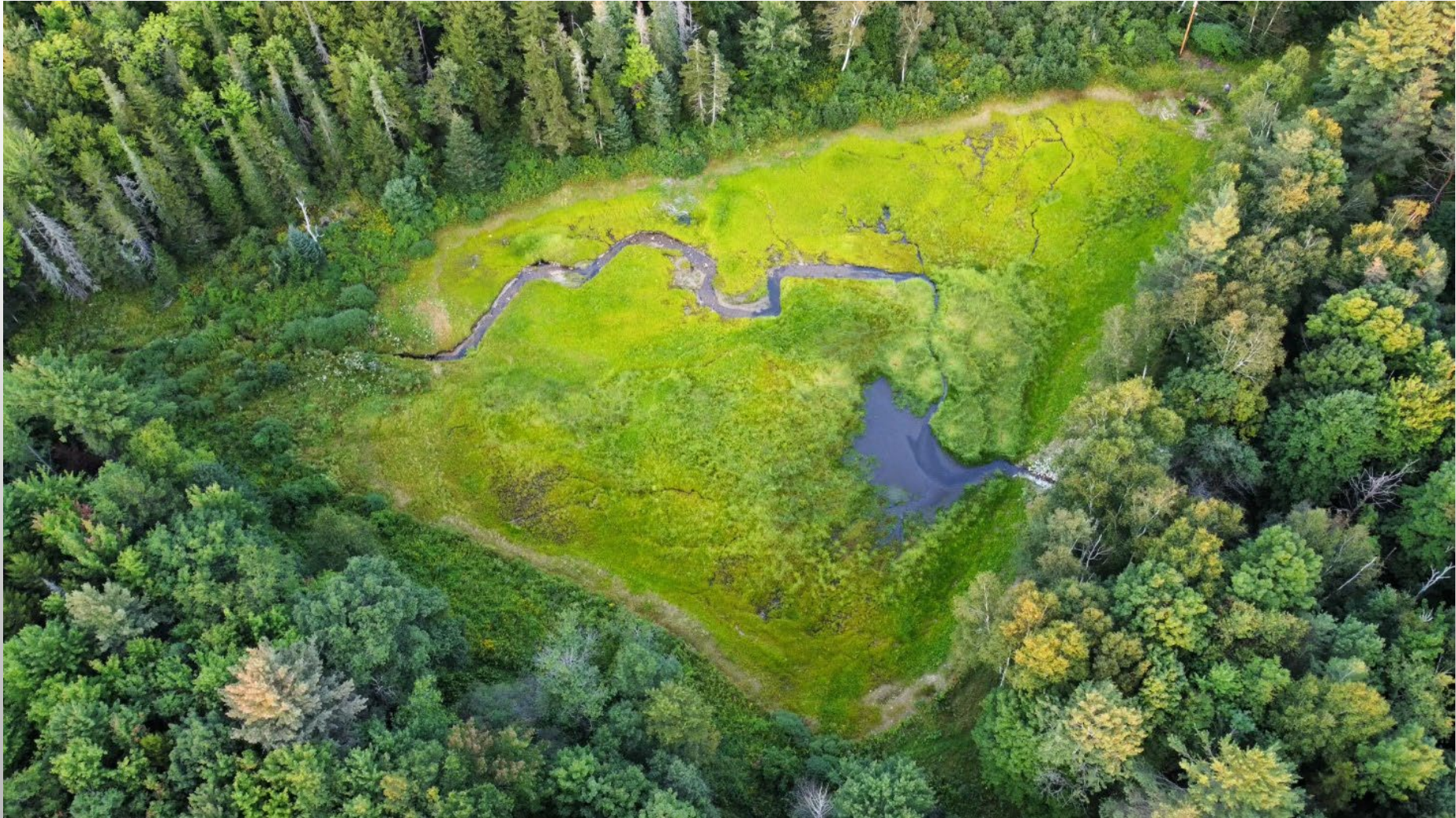
Connolly Pond Dam Removal, Photo by Marc Cimonetti
