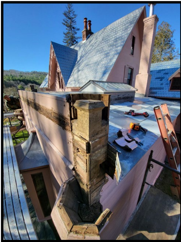
Crenellation Restoration, November 2022-May 2023
