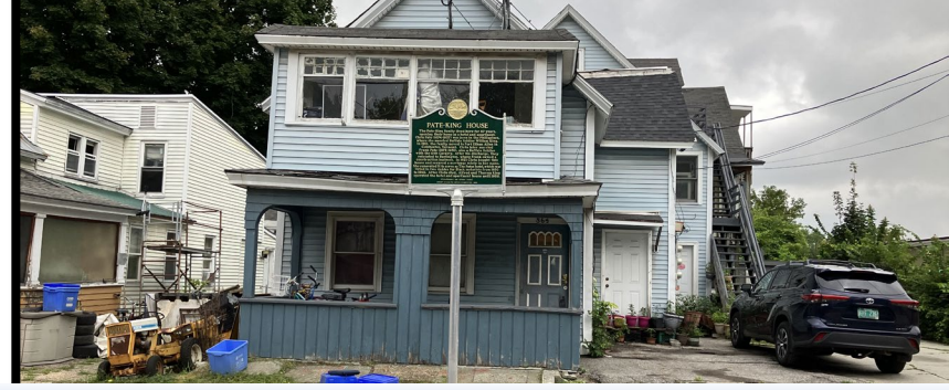
Pate-King House, Burlington – August 9, 2022 Installation
