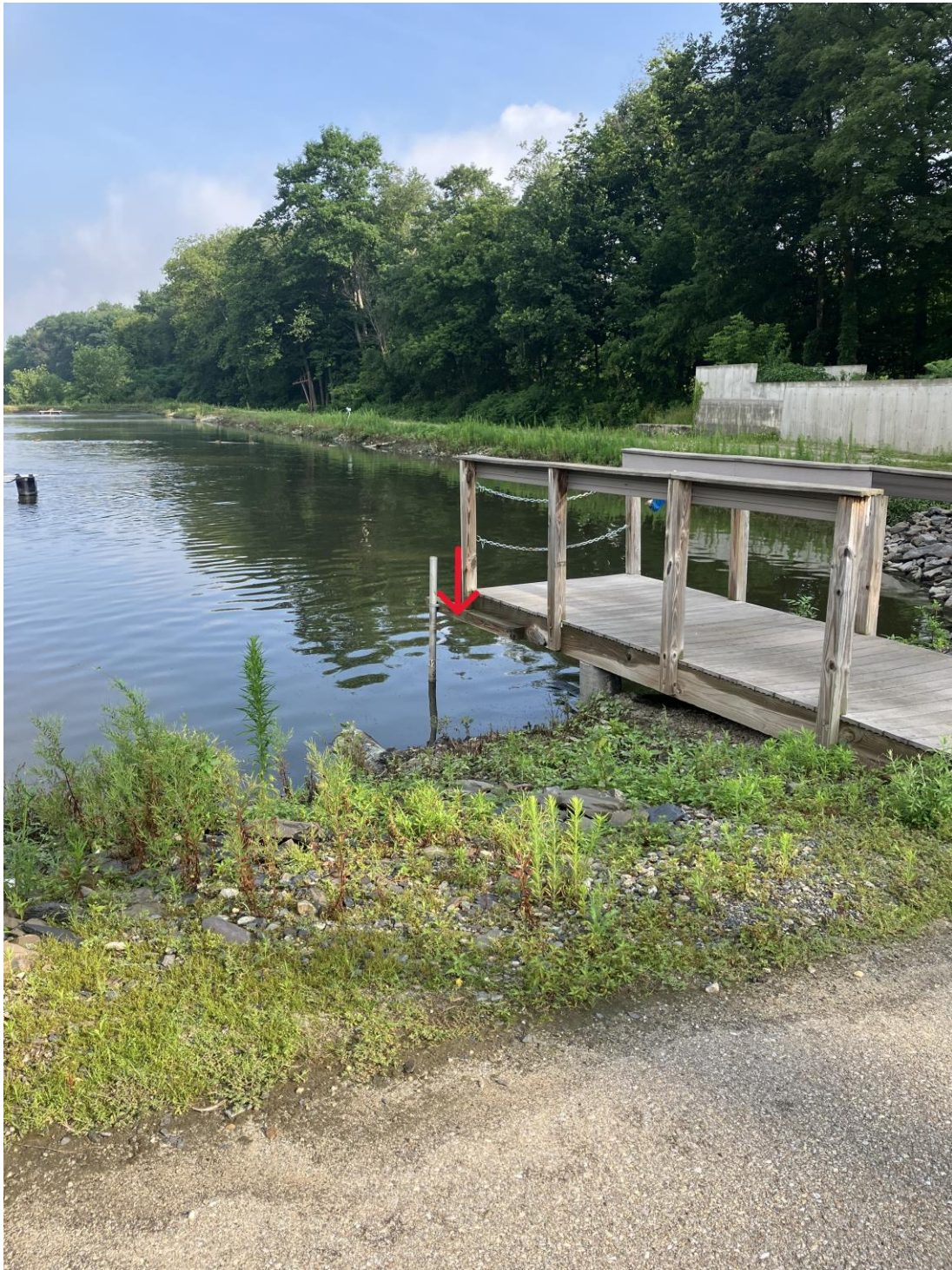
4- View of Lagoon Showing High Water Mark at Bottom of the Platform
