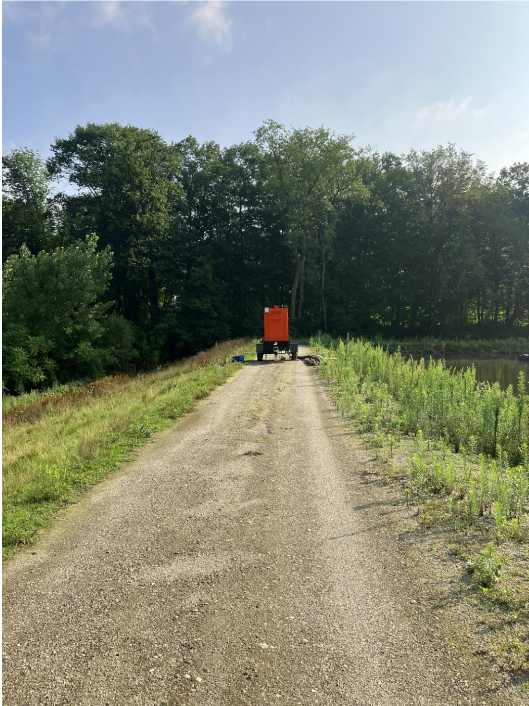
8- Godwin Pump Used to Pump Down Lagoon 1 During the Flood Event
