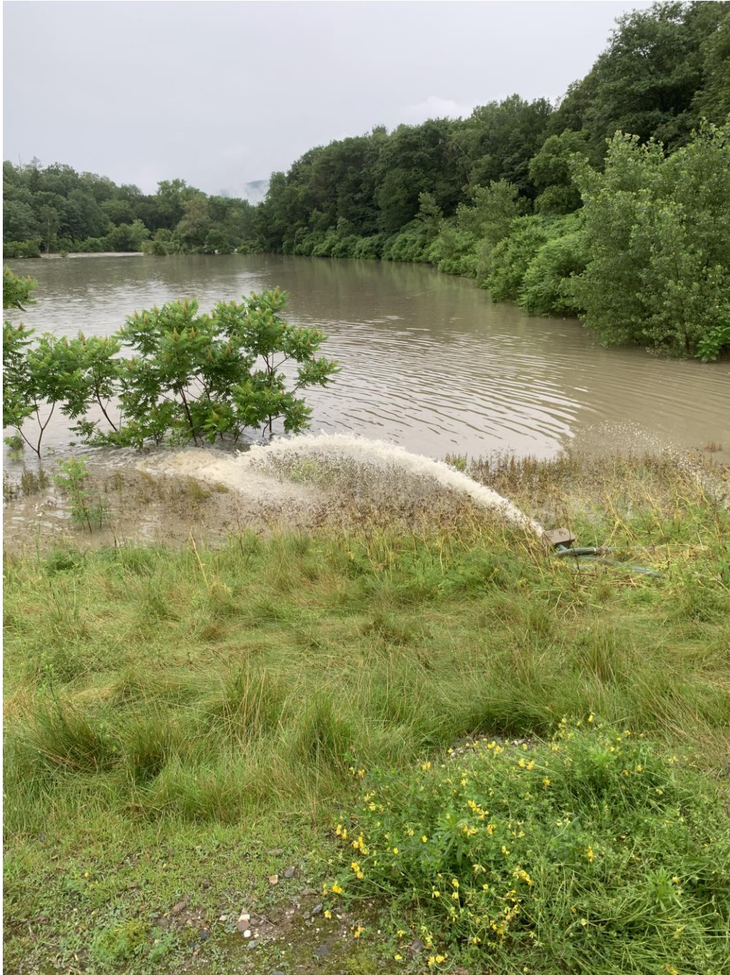
1- Water from Lagoon 1 Being Pumped By Godwin Pump Into Adjacent Field During the Flood Event (Photo courtesy of Chief Operator Matt Jones)
