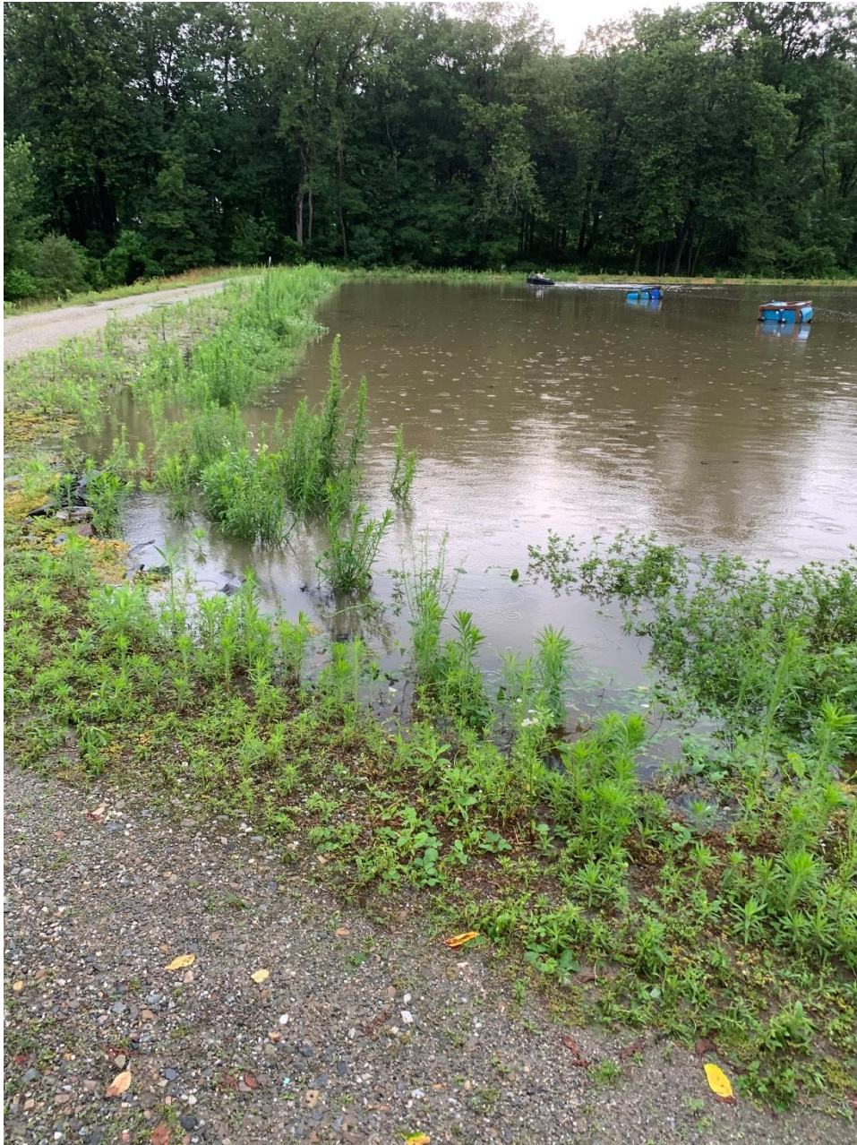
6- View of Backside of Lagoon 1 Prior to Installing the Godwin Pump During the Flood Event (Photo Courtesy of Chief Operator Matt Jones)
