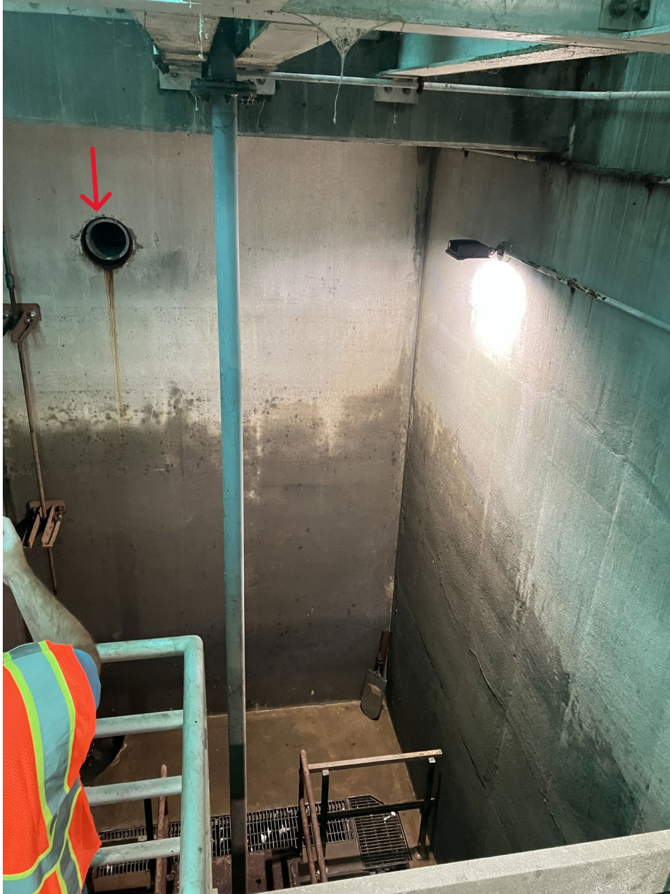
3- Main Pump Station Overflow Pipe Noted
