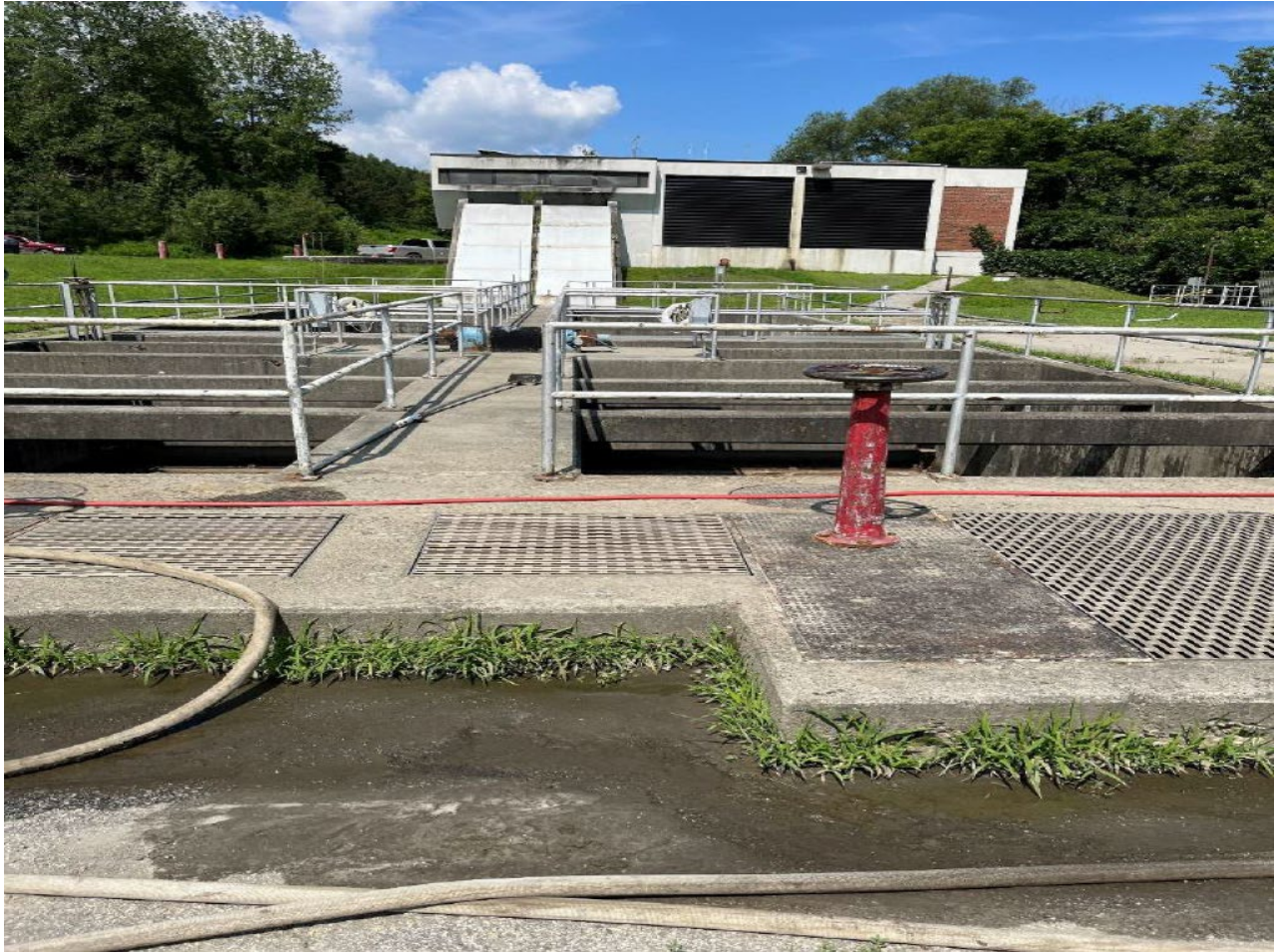
Primary clarifiers foreground, main plant building rear
