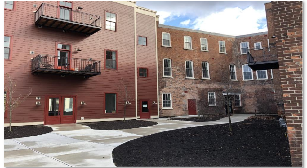
Completed Phase 1 of Putnam Block.
