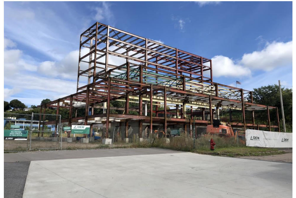
Partial demolition and site stabilization of the Moran Plant.
