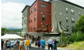
Village Center Apartments, Morrisville
