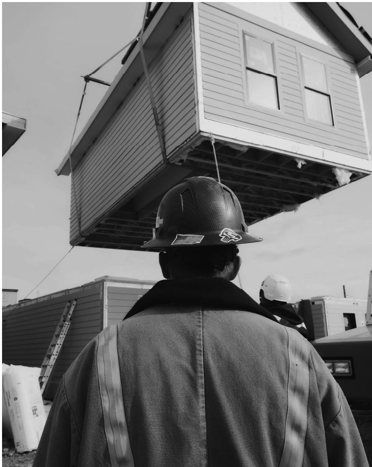
Cranes swing prefabricated housing units into place.
