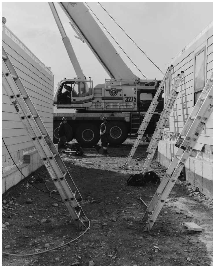
A crane being repositioned to build the next group of homes.
