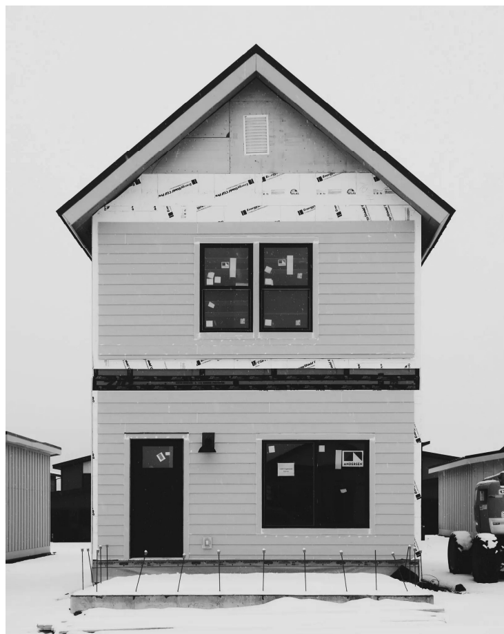
Snow falls on a Fading West modular home as it waits for finishing touches in Colorado.
