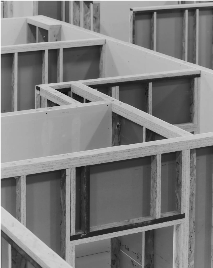
Fading West uses engineered lumber in its housing modules.
