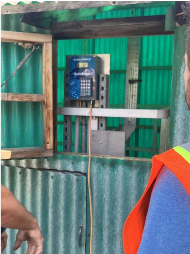
7- New Flow Meter with Temporary Wiring
