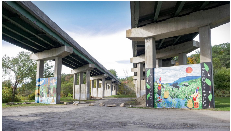
Montpelier artist Carolyn Shapiro and Abenaki "Missisquoi" artist Abena Songbird, with the assistance of many volunteers, completed two murals on I-89 bridge piers in Gateway Park in Montpelier, adjacent to U.S. Route 2 and the Winooski River. This is the first community-driven art installation completed through AOT's new art installation policy.
