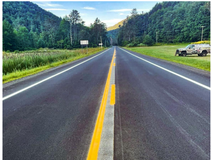
PLYMOUTH - BRIDGEWATER. It was a busy summer along VT Route 100 as crews completed 16 miles of paving, replaced guardrail, and installed rumble strips on the roadway.
