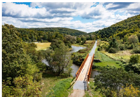
Completed LVRT bridge in Wolcott.
