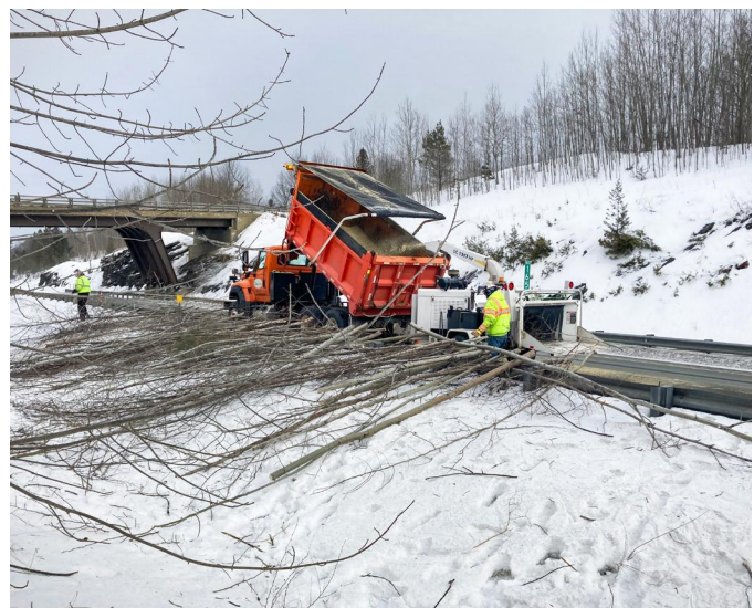
COVENTRY. When they aren't busy with their many winter-specific maintenance tasks, our crews work on other year-round tasks such as brush cutting to keep sightlines clear and safe on the roadway.
