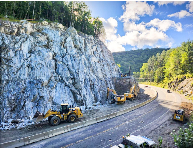
WOODFORD. A multi-year ledge stabilization project on VT Route 9 was largely completed in 2022. The rockface was cut 30 feet back from the roadway, improving sight distances and safety from potential rock falls.
