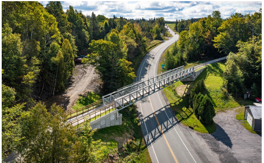
A new rail trail bridge was installed over VT Route 15 to connect segments of the LVRT in Walden.
