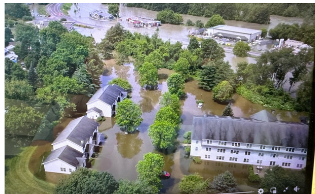
Mann's Meadow Family Apartments (left.) Mann's Meadow Senior Apartments (right) was relatively unscathed.
