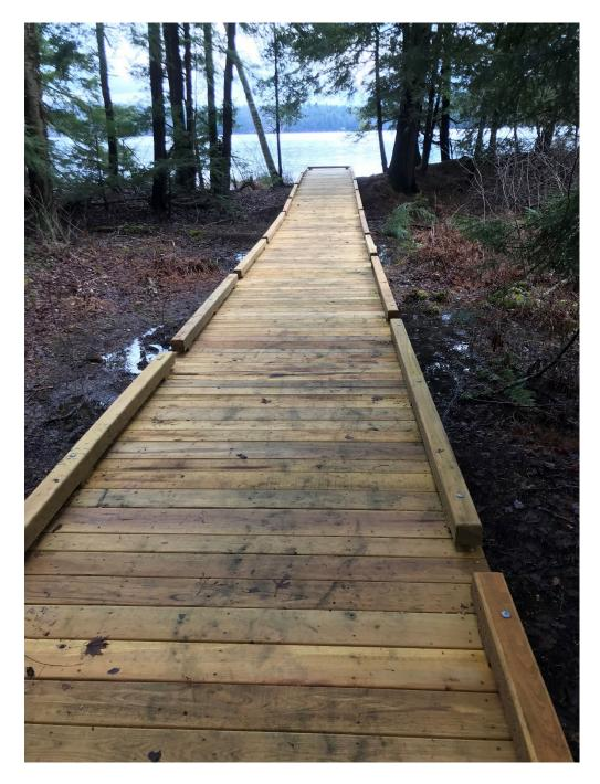
Figure 2. Sunset Lake (Benson) – This boardwalk is part of a newly constructed ADA accessible access area that was constructed on the north side of Sunset Lake. The project included significant upgrades to a camp road that leads to a new parking area which will serve both the fishing access area and Pond Woods Wildlife Management Area. From the parking area, there is a short gravel trail which leads to the boardwalk and lake shore where anglers and paddlers can access the lake.
