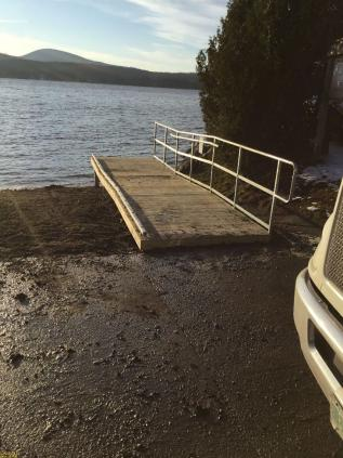
Figure 1. New accessible dock abutments were installed at the Marshfield Reservoir Access Area/Mollys Falls State Park in Cabot (top) and Lake Willoughby Access Area in Westmore (bottom) this past November. Both docks will be fully accessible and enhance boating access to these popular waterbodies.
