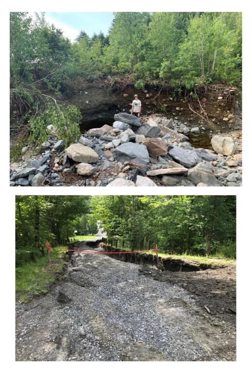
Figure 3. Storm damaged facilities – Gale Meadows Dam (top) suffered a significant washout as water overtopped the auxiliary spillway and eroded much of the large boulders. Rood Pond's (bottom) access road was washed out due to an undersized culvert under a town road. Debris was deposited on the boat ramp and in adjacent areas in the pond.
