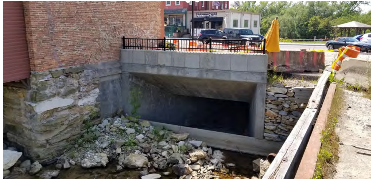
Center Street Overflow Culvert
