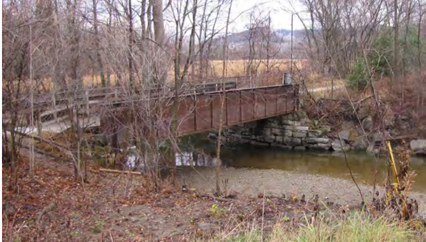
Original Trail Bridge
