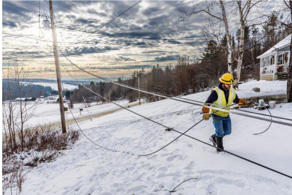
Washington Electric Co-op lineman Donnie Singleton carries part of a downed and de-energized power line, getting ready to splice it. – John Lazenby, The Bridge
