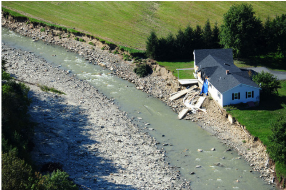
Extensive erosion damaging a home along Route 11 outside of Chester, VT. Photo Credit: www.mansfieldheliflight.com/flood/
