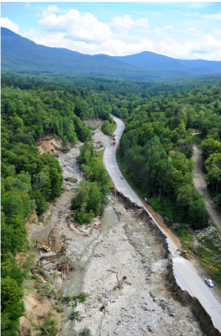
Severe damage to Vermont Route 4 in Killington, VT due to fluvial erosion during Tropical Storm Irene
