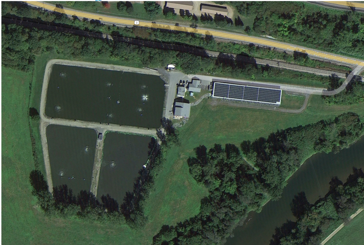
Waterbury VT WWTF (Image Courtesy Google Earth)
