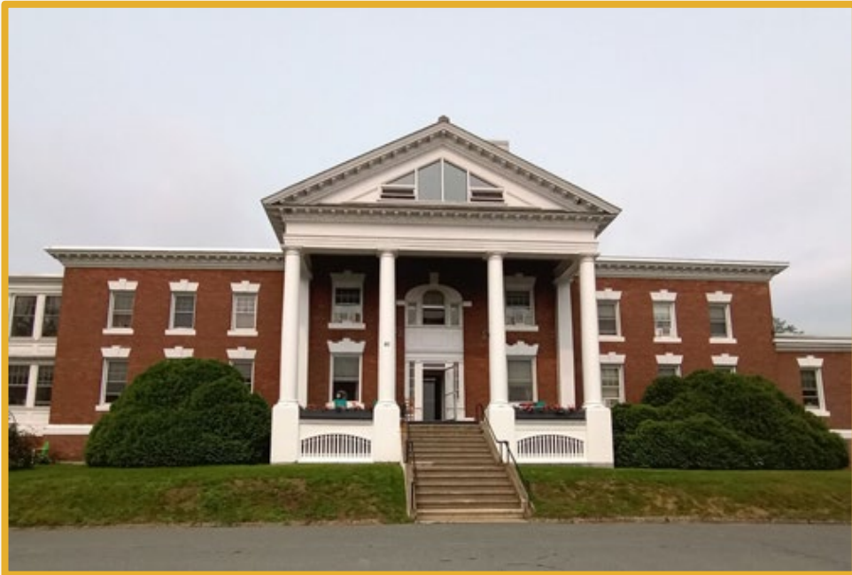
Brightlook Apartments St. Johnsbury | 18 units
