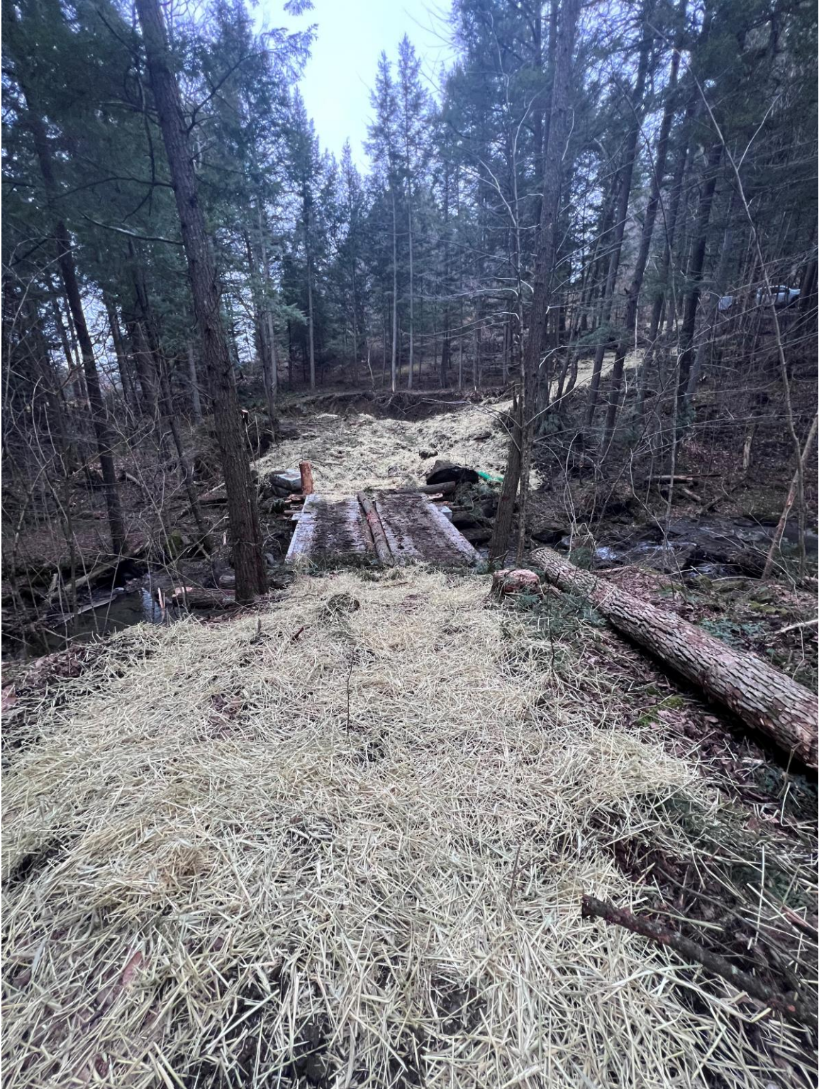
Temporary skidder bridge installation
