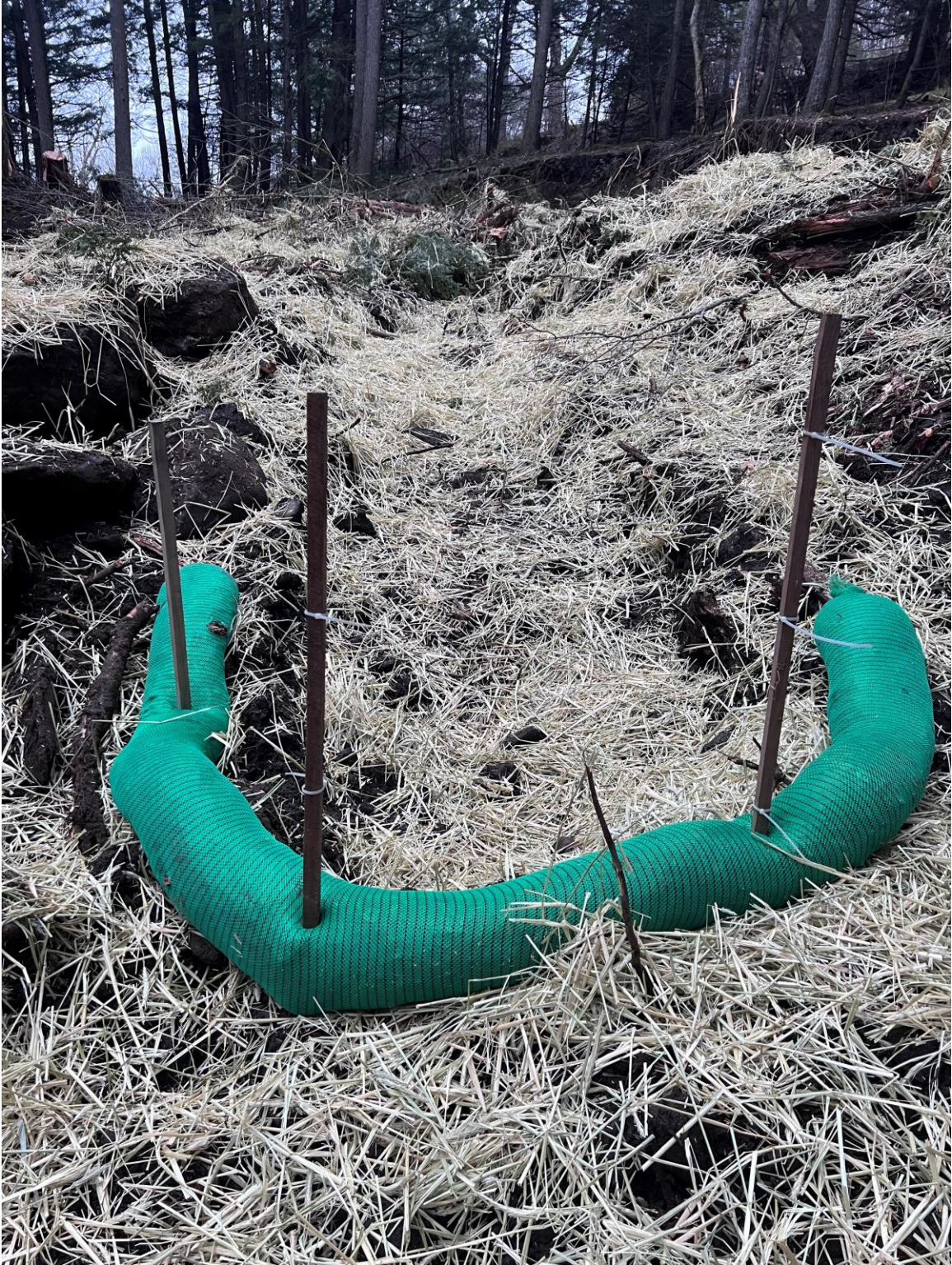
Filter sock installed at the outlet of a ditch
