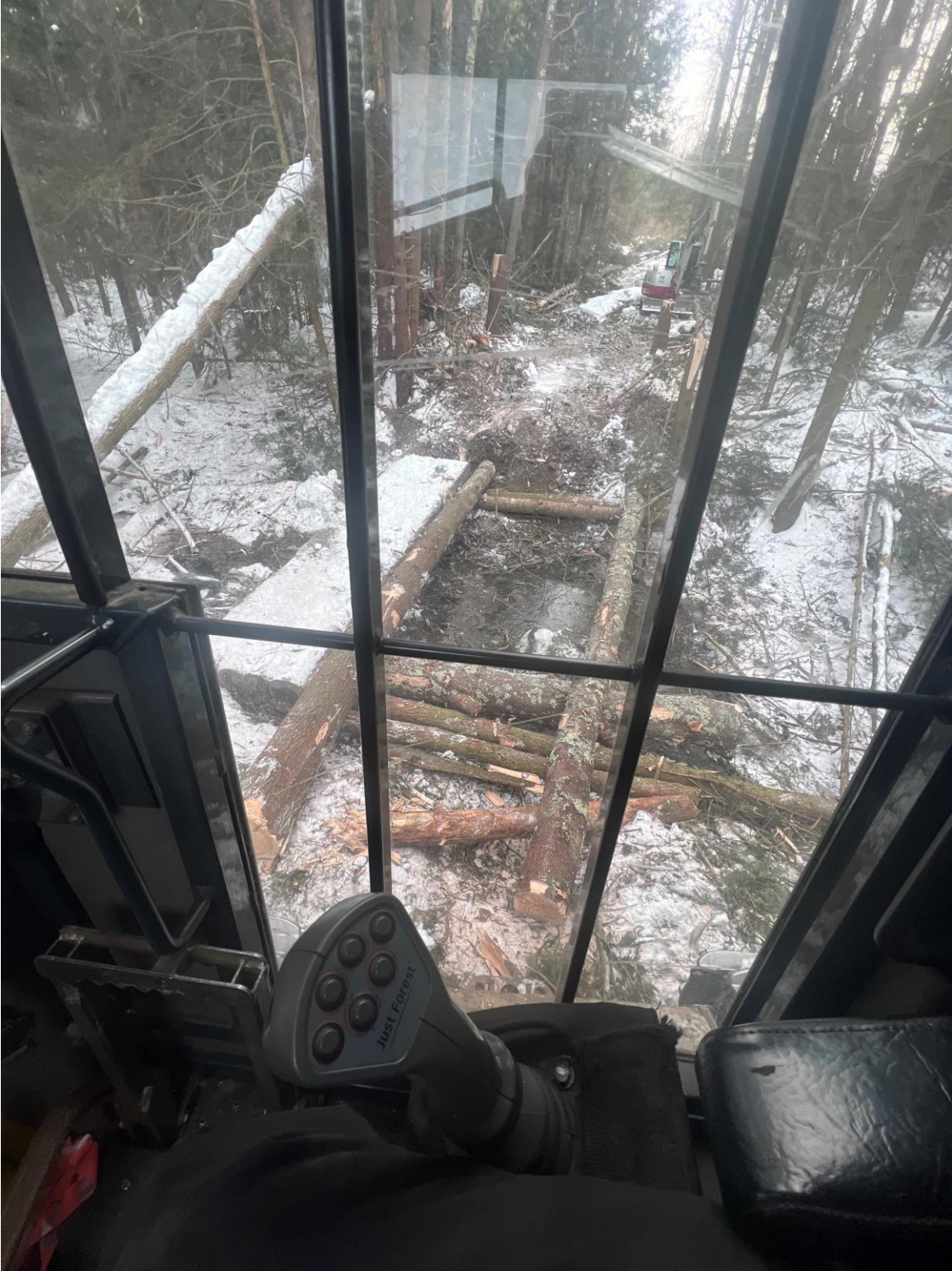
Installation of a temporary wooden skidder bridge on a stream crossing
