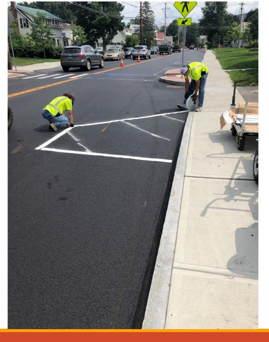
Durable pavement markings being installed concurrent with paving operations.
