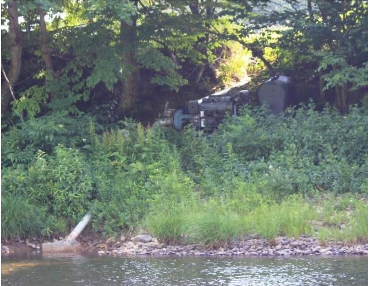
Figure 1: A surface-water diversion intake pipe and pump operation on Southern Vermont's West River near the Town of Newfane during low-water drought conditions of Summer 2020. Photo by David L. Deen, Connecticut River Valley Chapter of Trout Unlimited, 2020.
