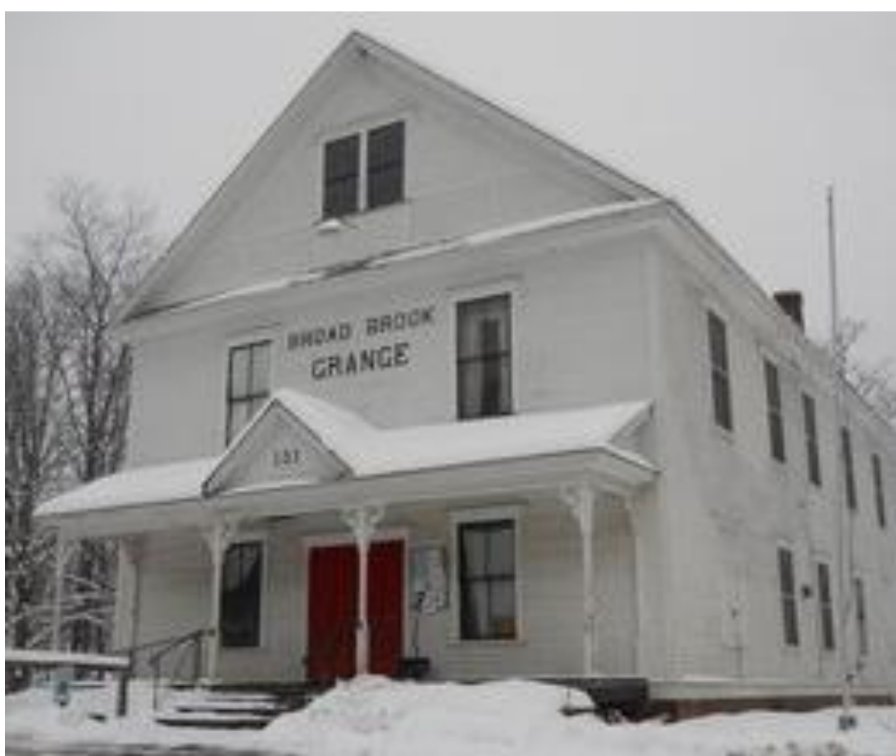
Broad Brook Community Center, Guilford
