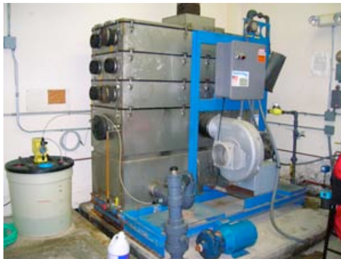
State-owned "air stripper" removes MTBE and other gasoline contaminants from mobile home park water
