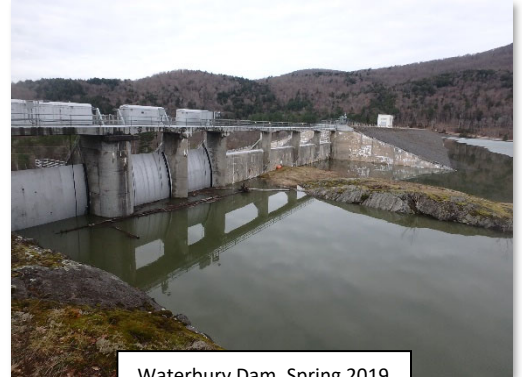
Waterbury Dam, Spring 2019
