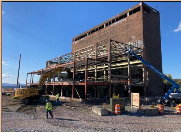
Start of demolition and site stabilization of the Moran Plant.
