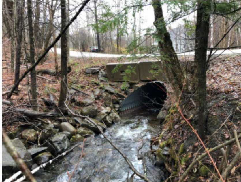
Infrastructure resiliency project in Thetford
