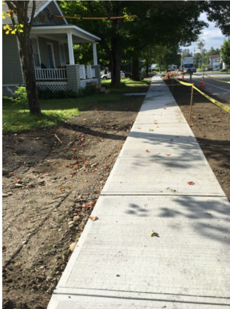
Sidewalk construction in Underhill
