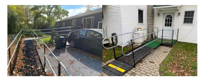
VCIL uses modular ramps which can be moved and retrofitted for use in a new location if the peer moves; the ramps can also be moved to a new location if the peer no longer needs the ramp.
