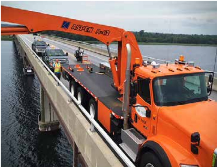
GRAND ISLE. VTrans staff inspect a bridge in the Champlain Islands
