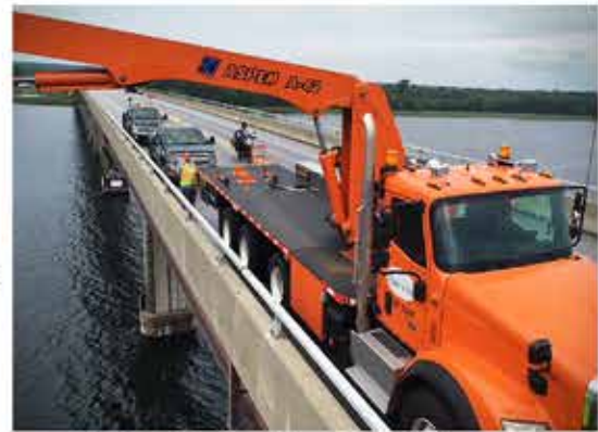
GRAND ISLE, VTrans staff inspect a bridge in the Champlain Islands
