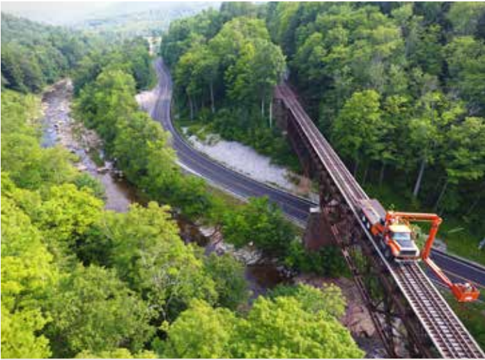
CUTTINGSVILLE. A crew from the VTrans Rail section performs a bridge inspection using a specialized “snooper” truck. The photo was captured by the Agency’s new aviation drone.
