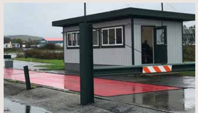
FAIR HAVEN SCALE REPLACEMENT. The existing failed platform scale at the Fair Haven Scale House was replaced by a brand new, state of the art enforcement platform scale. The new scale enhances Vermont's Size & Weight Enforcement Plan with the Federal Highway Administration and allows DMV Enforcement Officers to more easily ensure vehicles are in compliance with weight limits.
