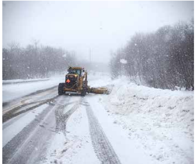
With excess amounts of snow, VTrans crews “wing back” snow mounds on the roadside to make room for the next big storm.
