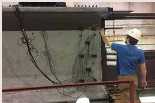
EXPLORING THE POTENTIAL FOR ACOUSTIC EMISSION SENSING TO INCREASE BRIDGE LIFE Researchers are determining whether Acoustic Emission (AE) testing can be applied to Quality Assurance/Quality Control efforts. AE has the potential to increase the service life of bridges by identifying the level of cracking in prefabricated reinforced concrete elements.
