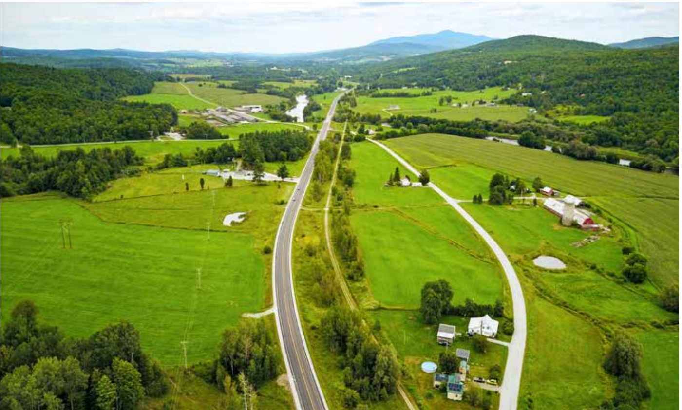
RICHFORD. Resurfacing of VT-105A along a 2-mile stretch from Richford to the Canadian Border.
