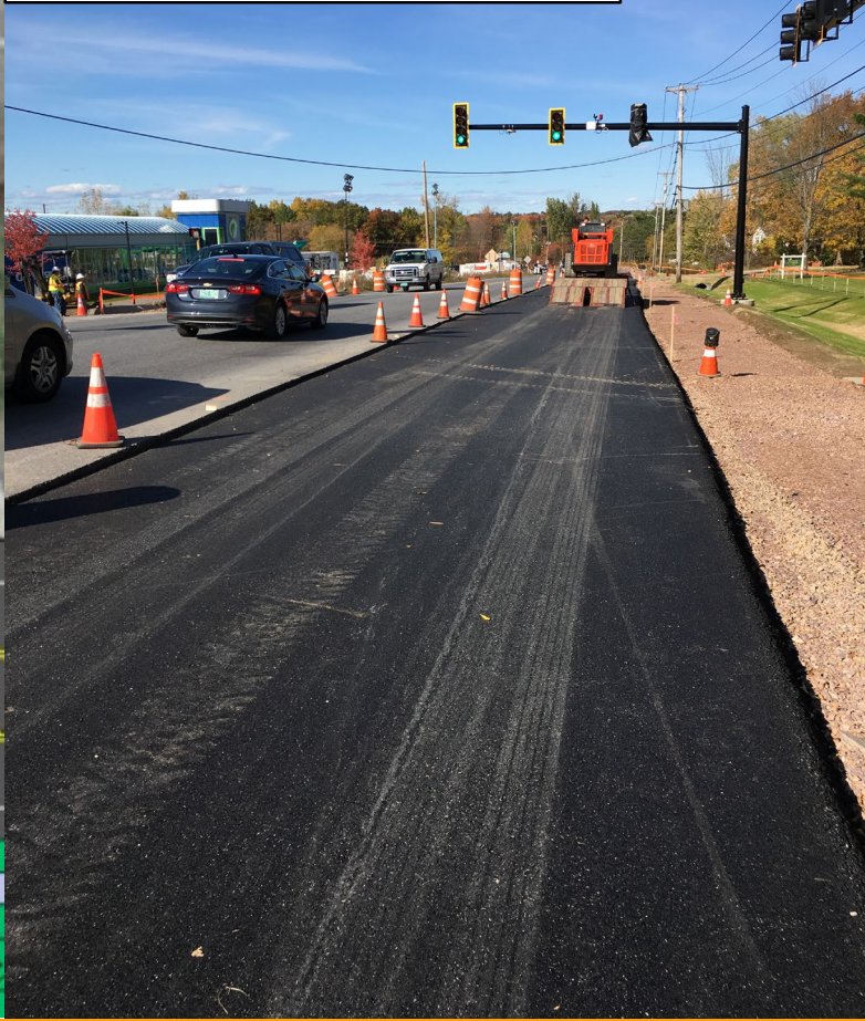
VT ROUTE 2A - WIDENED
