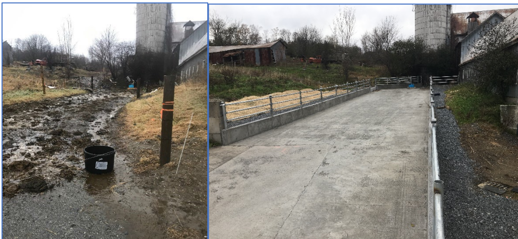
From left to right, before and after photos show clean water diversion and heavy use area protection.
