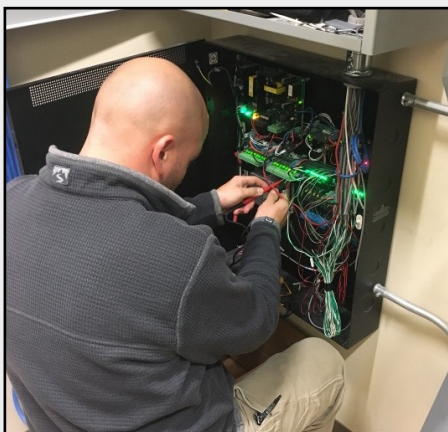
Left: An Electronic Security Systems Technician conducts maintenance on a card access system.
