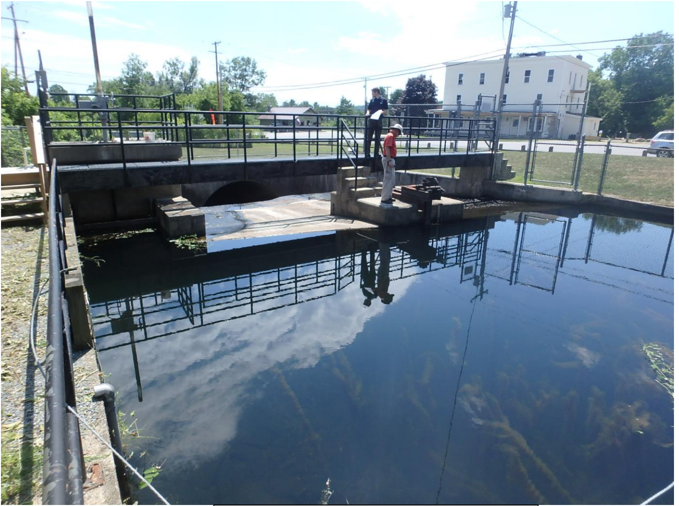
Photo 9: Lake Bomoseen Dam, minor repairs.
