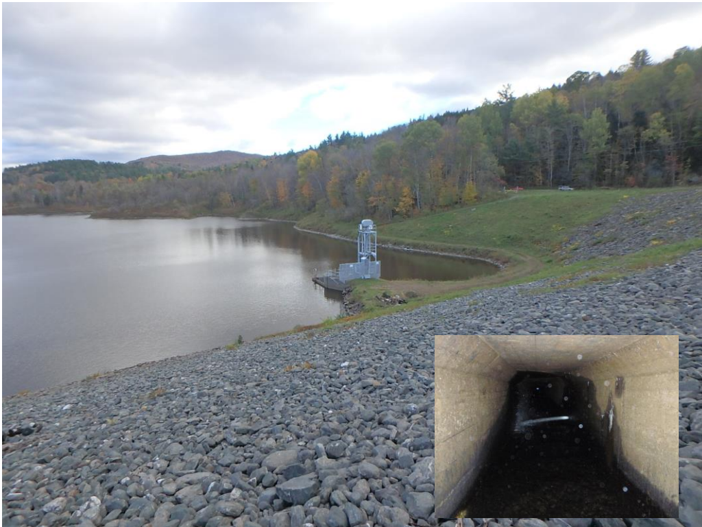
Photo 5: Wrightsville Dam, principal spillway intake structure and leak in spillway tunnel.
