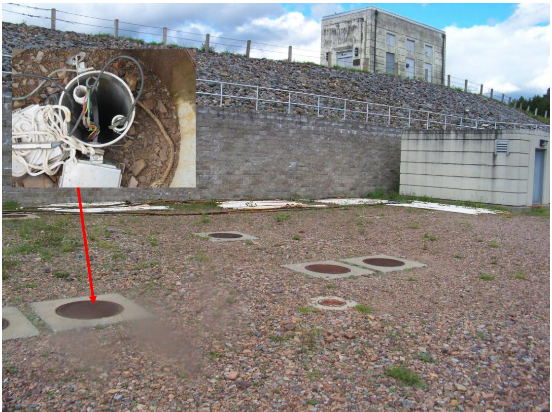
Photo 4: Waterbury Dam Seepage Collection System.
