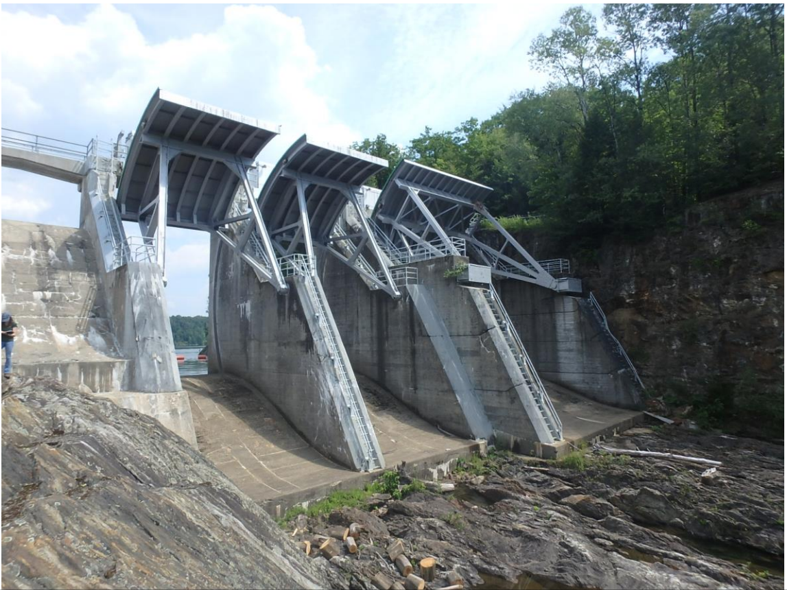
Photo 3: Waterbury Dam Spillway, the access ladders requiring a fall protection system can be seen.
