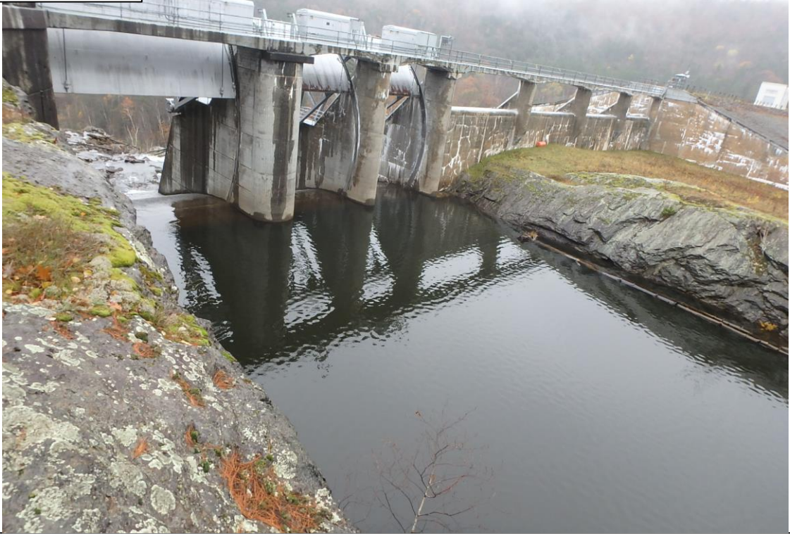
Photo 1: Waterbury Dam Spillway Replacement, Risk Assessment, $215k from previous years. The approach channel in need of a new boat barrier can be seen.
