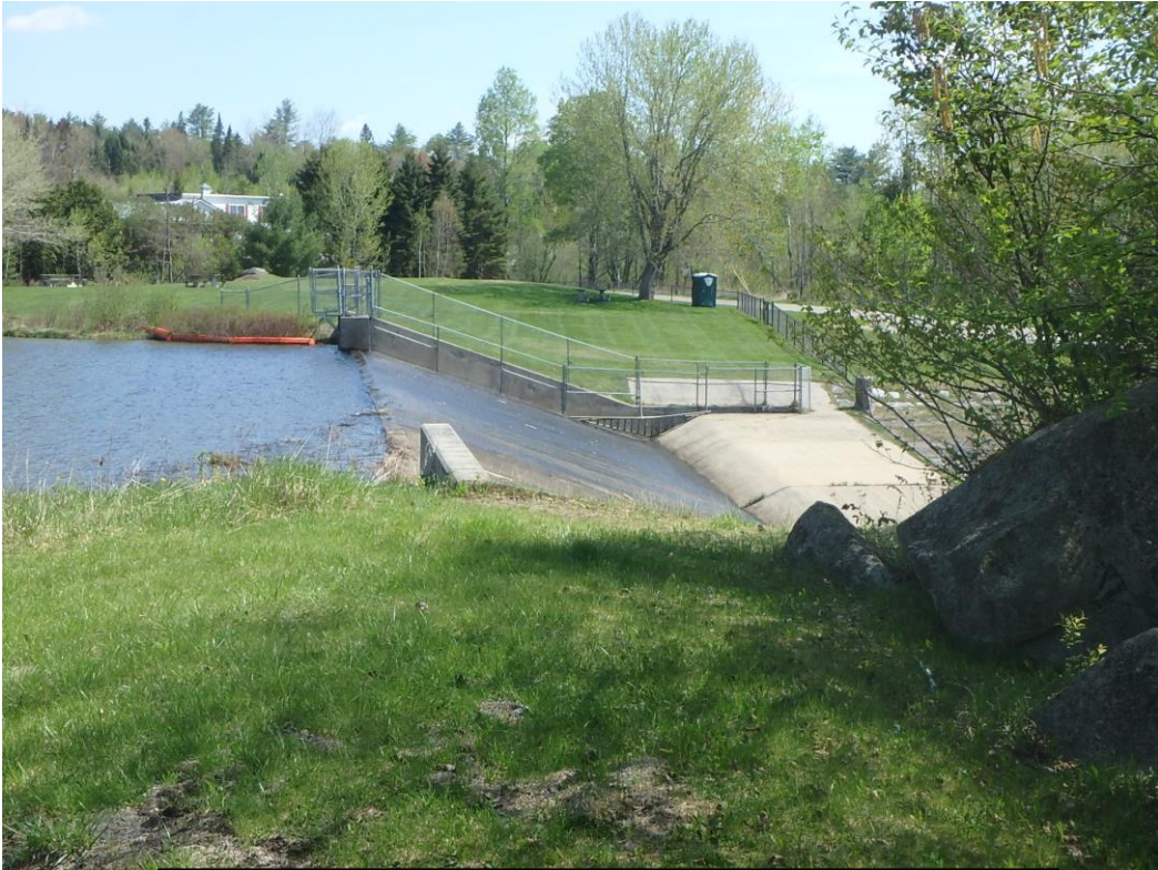
Photo 7: Miles Pond Dam, various minor repairs needed.
