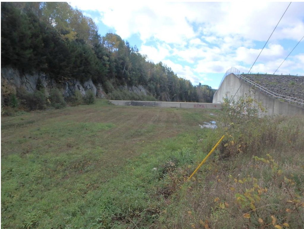
Photo 6: Wrightsville Dam, aux. spillway, note overgrown and aging rock cut at left side of image.
