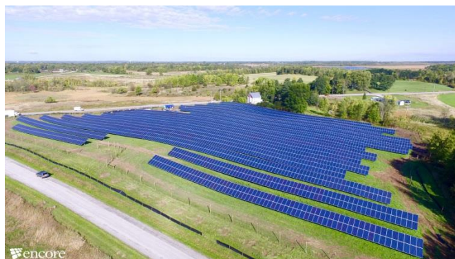
Alburgh Project (Photo credit: Encore Renewable Energy)
