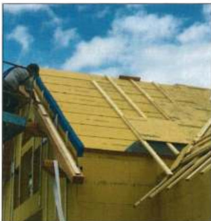
Notice the air layer being created between the sheathings
