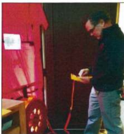
Using a blower door to determine amount of air leakage
