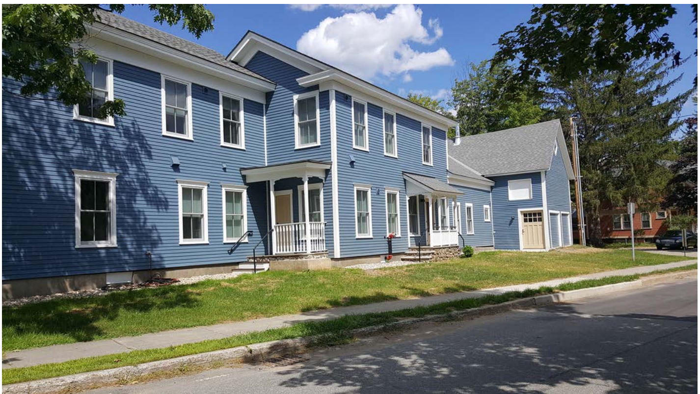
▲ Above: Clara Martin Center staff in front of the recently rehabilitated, historic building, that now provides four homes with support services for residents with chronic mental illness plus office and program space for the Clara Martin Center.
