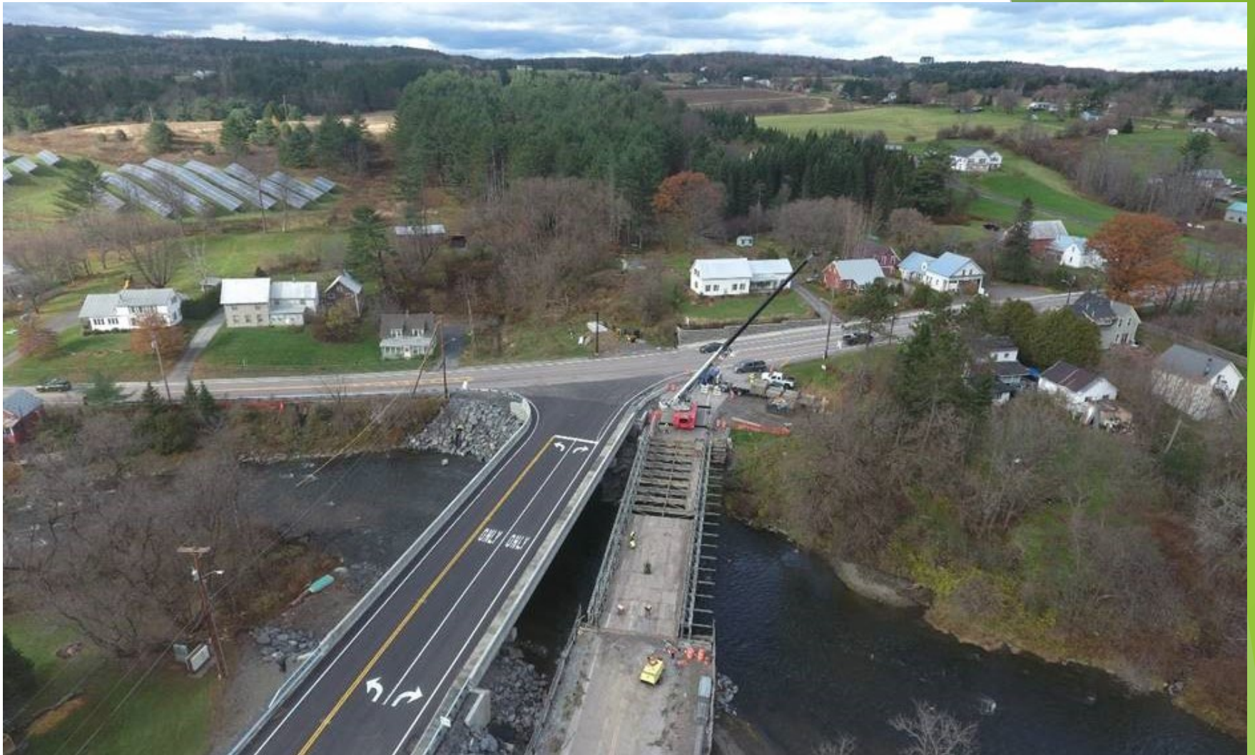
East Montpelier Route 14 Bridge over Winooski River
